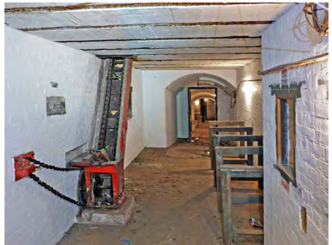
Devil's Gap Battery: magazines and shell lift
